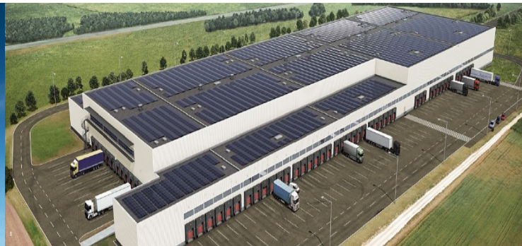
GE Hybridkraftwerk Power Conversion Berlin Marienfelde Tomorrow is made in Europe
